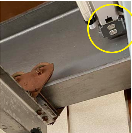
observed existing electricity supply at ceiling system will supply electricity to the movable rods via coiled extension cords with magnetic power strips. These power supplies can thus be moved to along the beam according to the configuration of the rods. The nature of the I beams will keep the wiring concealed along the lower interior half of the beam, not visible from the ground.
